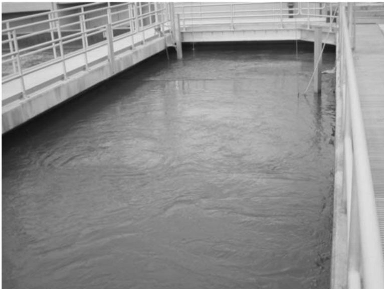
FIGURE 5.24 Surface of anoxic zones in Southwest plant, Jacksonville, Florida.
