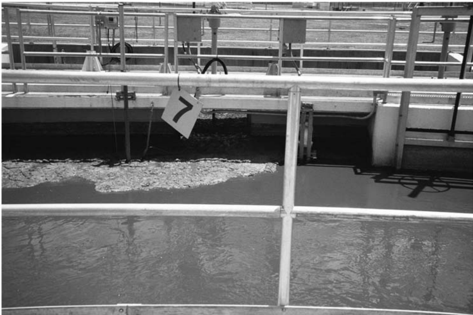
FIGURE 9.9 South Cary Water Reclamation Facility sidestream RAS fermentation zone.
