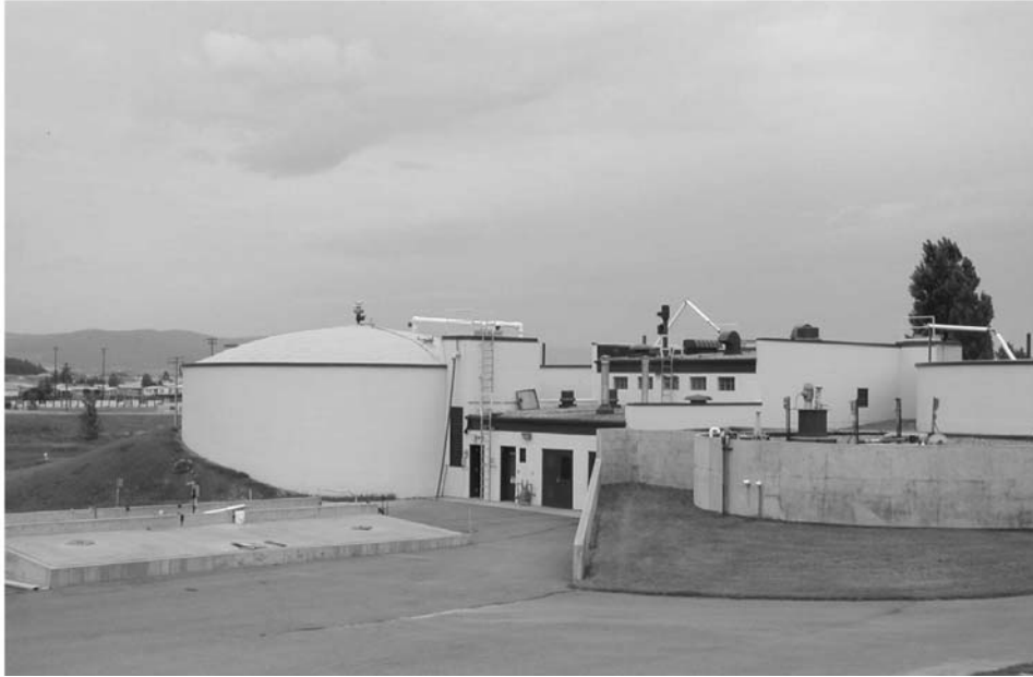
FIGURE 9.11 Kalispell complete-mix fermenter and thickener.
